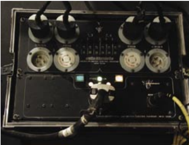
Figure 10. Checking phase (chain direction)
